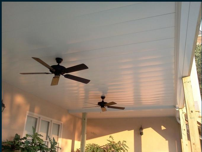
The underdeck system is designed so that any particular panel may be removed without disturbing the adjacent panels. It is an all aluminum construction.
